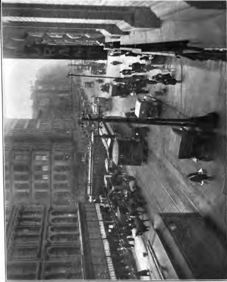
Illustration No. 5. —Washington avenue has a width of 80 feet in the business section. It typifies the minimum width major traffic street with trolley line as suggested in this report.
